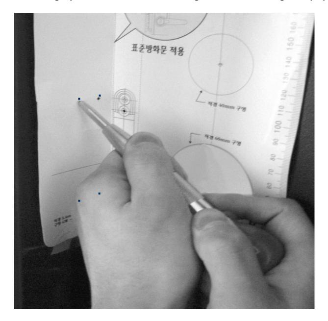
3. Marking 4points for lock strike using the Installation guide paper.
