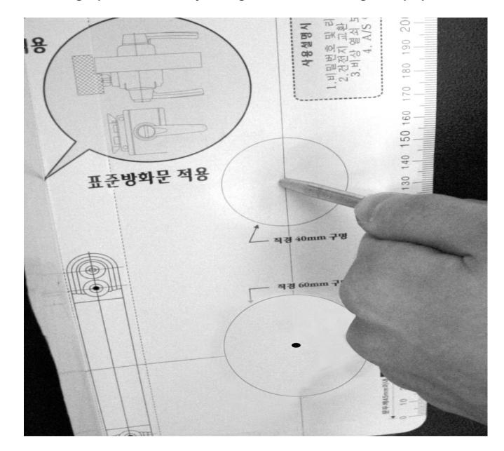
2. Marking 4points for body using the installation guide paper.
