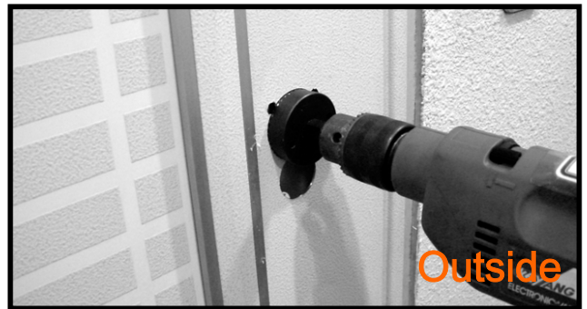
6. At first, Piercing 35mm's Hole at outside in the same location between Inside & Outside, then pierce 50mm's hole (outside only)
